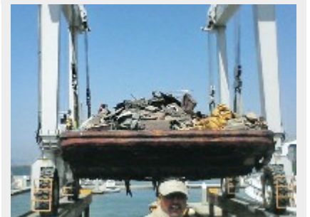
Boatyard manager Todd Roberts said his company's primary role in the project was to hoist debris from the barge and place it into containers. "We filled 17 dumpsters that held six tons of debris each," he said.
